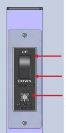
Press and hold the top of the rocker switch to call or send the lift up.
